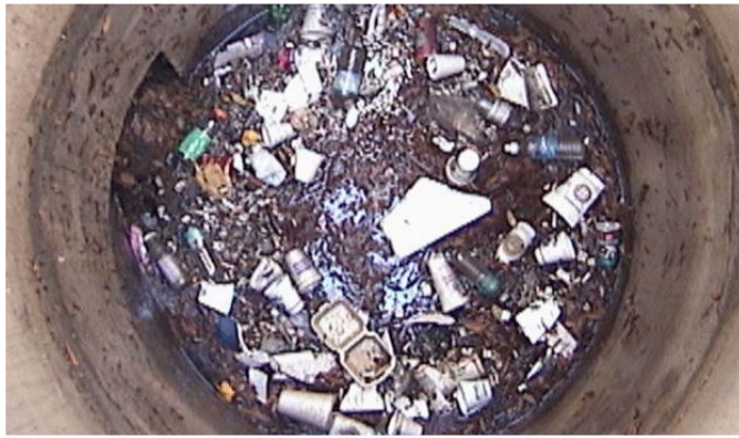
CDS provides trash control.
