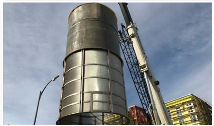
CDS standalone system removes trash and sediment.
