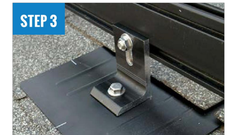
ATTACH L-FOOT TO RAIL
