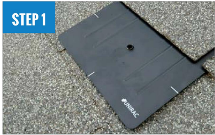
STEP 1 INSTALL FLASHKIT PRO FLASHING
