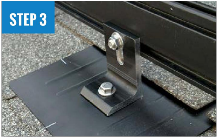
STEP 3 ATTACH L-FOOT TO RAIL
