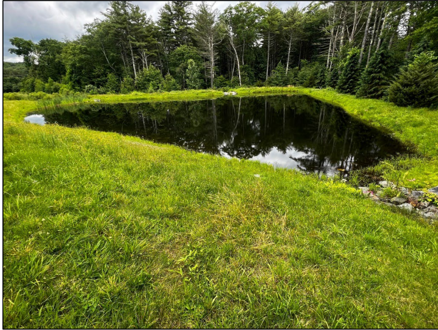
Photo 1: View of easternmost stormwater pond looking north.
