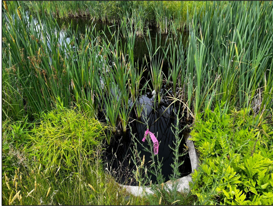
Photo 3: Culvert outlet to second pond. Note dense emergent vegetation (cattails).
