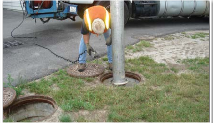
Most CDS units can easily be cleaned in 30 minutes.
