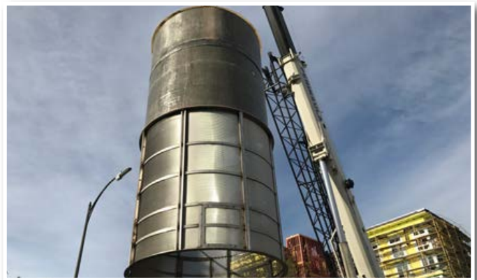
CDS standalone system removes trash and sediment.
