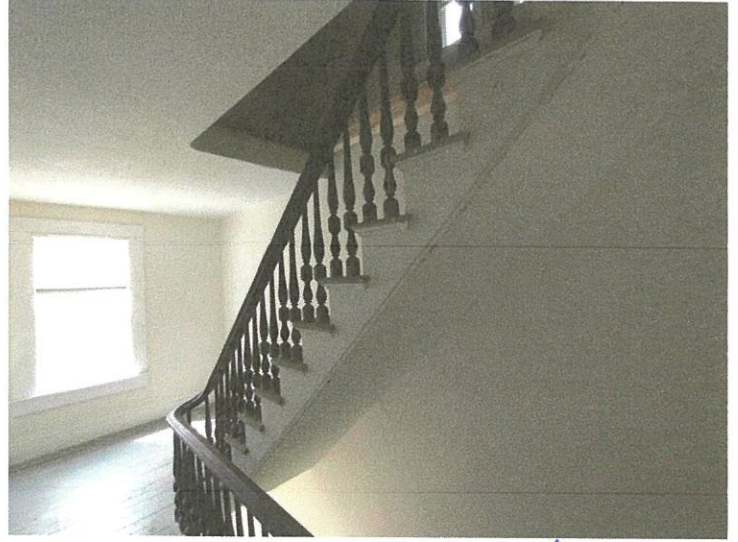
from 2nd Floor Landing
