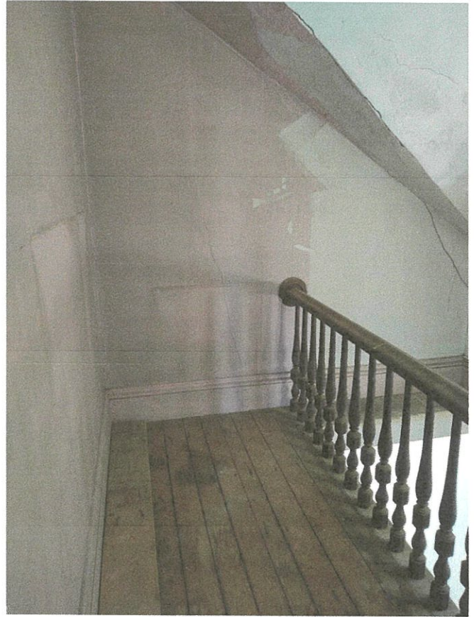
3rd Floor Landing
