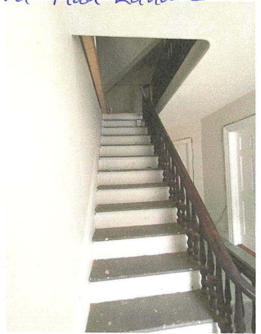
Stairs to 3rd Floor Landing
