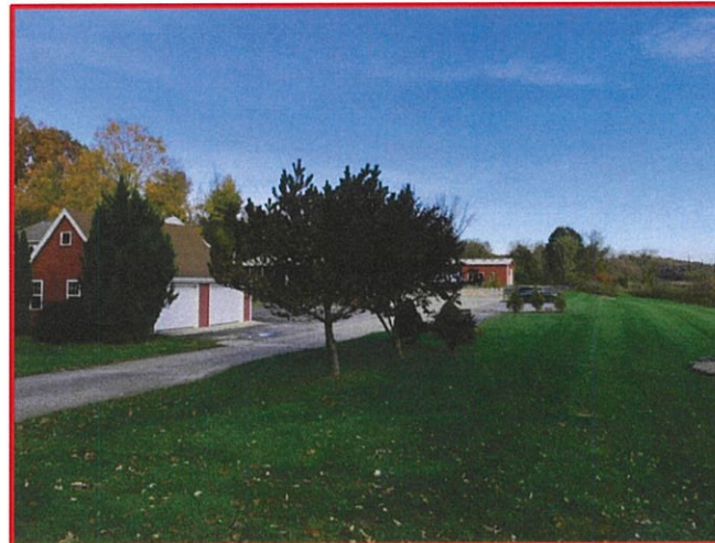
Road view of Building #3, #1, & #2
