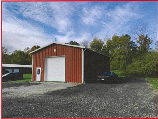
Building #2 – Front View
