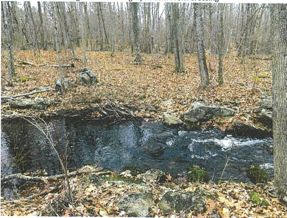
Figure 3 – View of Crossing Facing North
