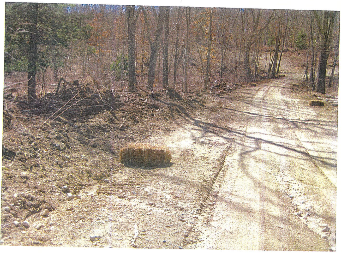
road widened near stream crossing on South side
