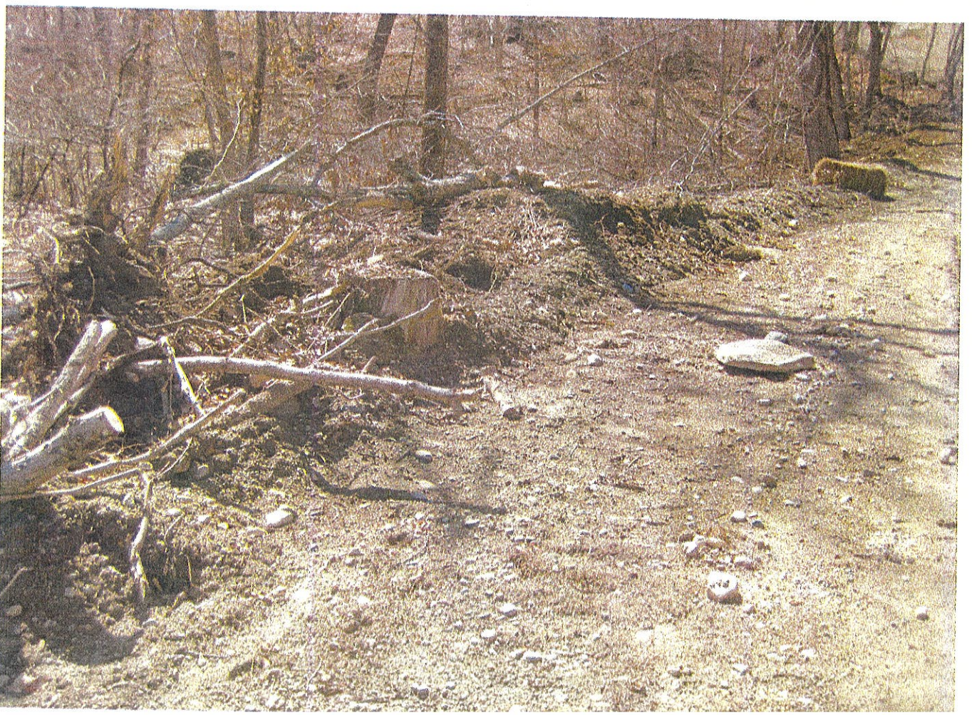
Access road widened at existing stream crossing,
