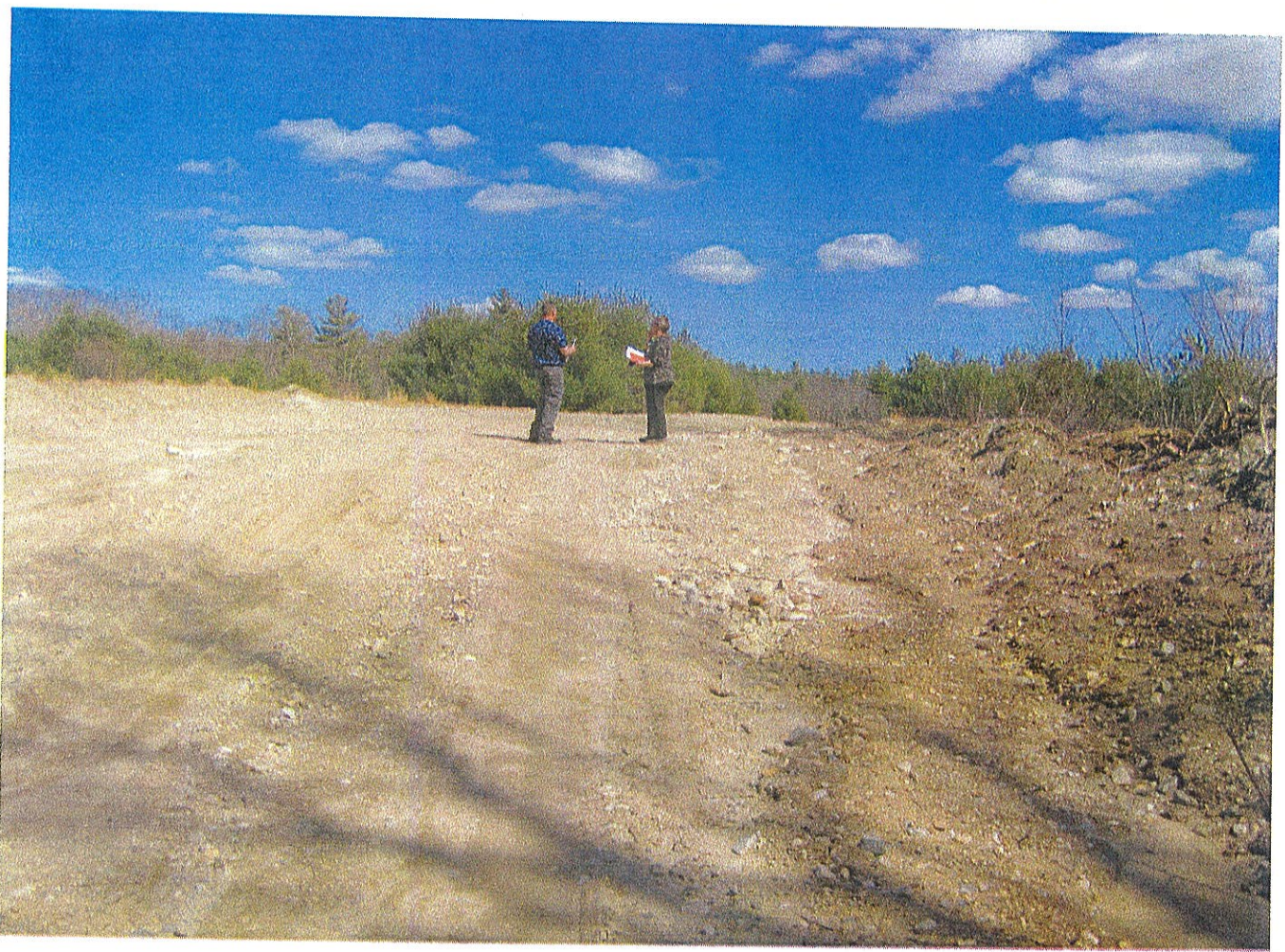
Road widened East of existing stream crossing.
