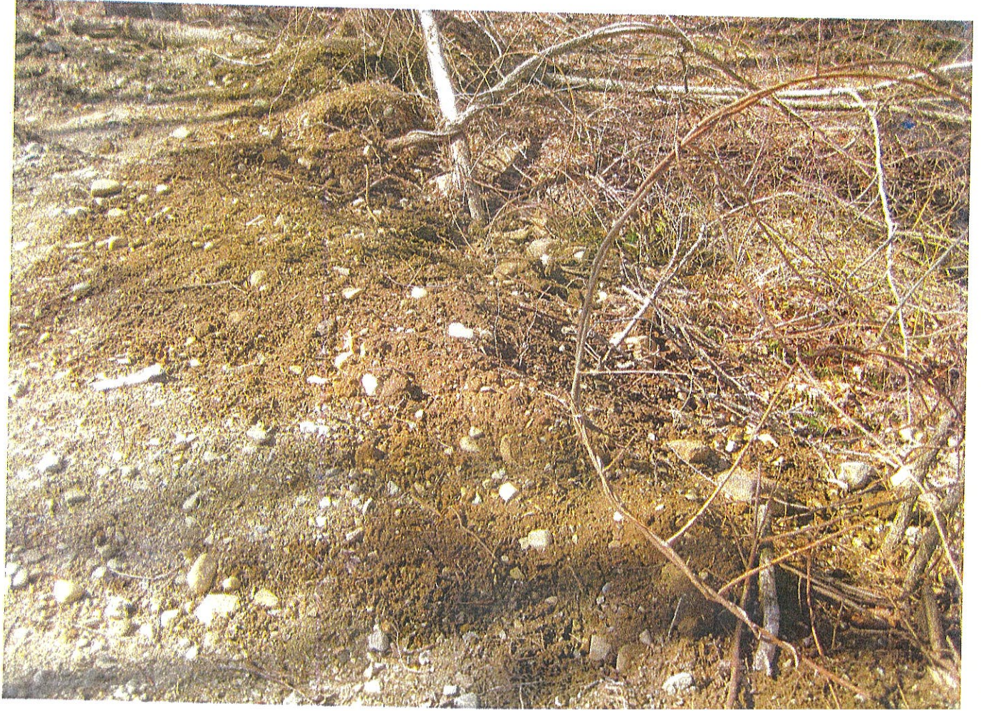
Fill on Northside of existing stream crossing.
