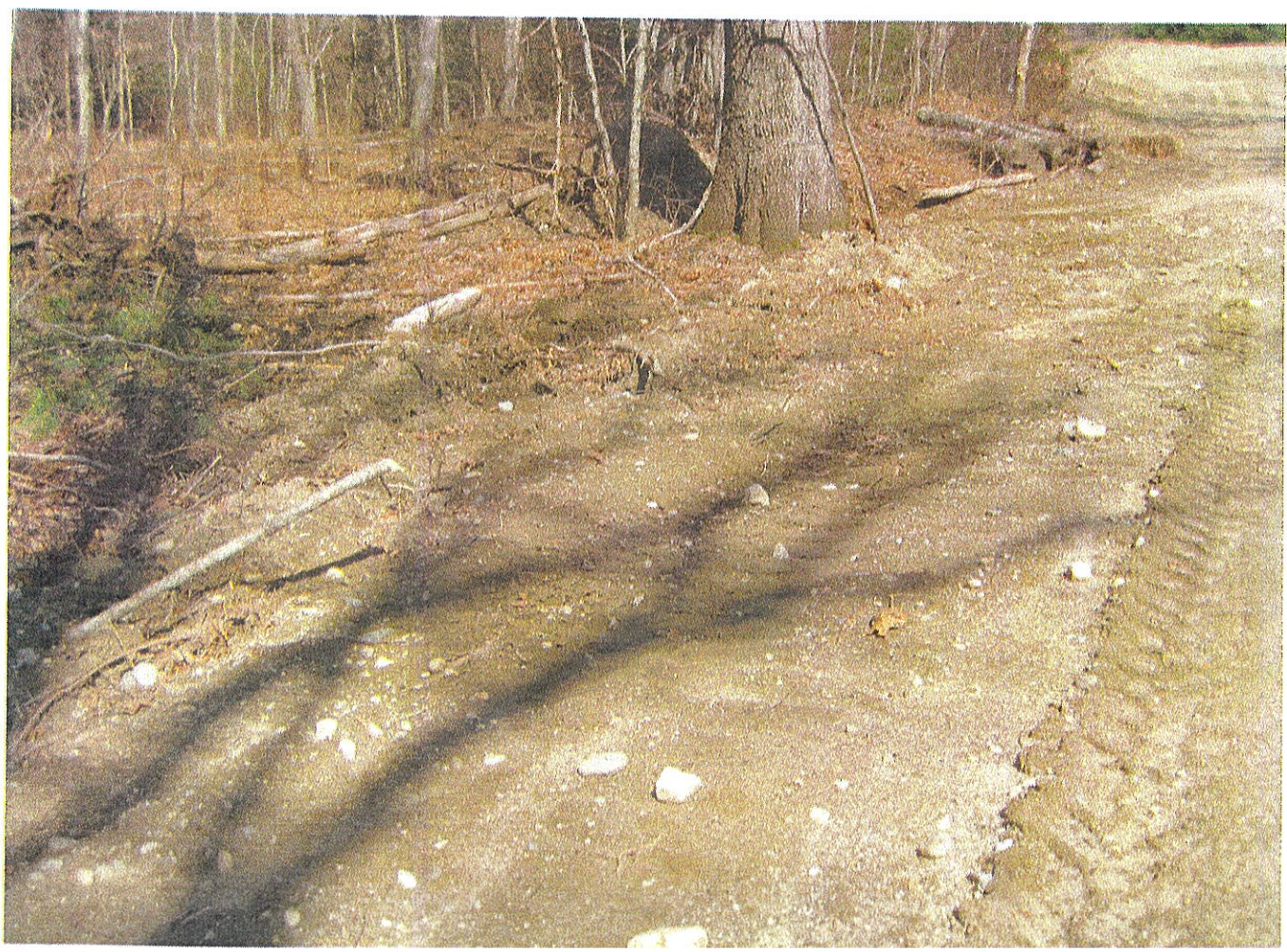
Road widened near stream crossing on North side.
