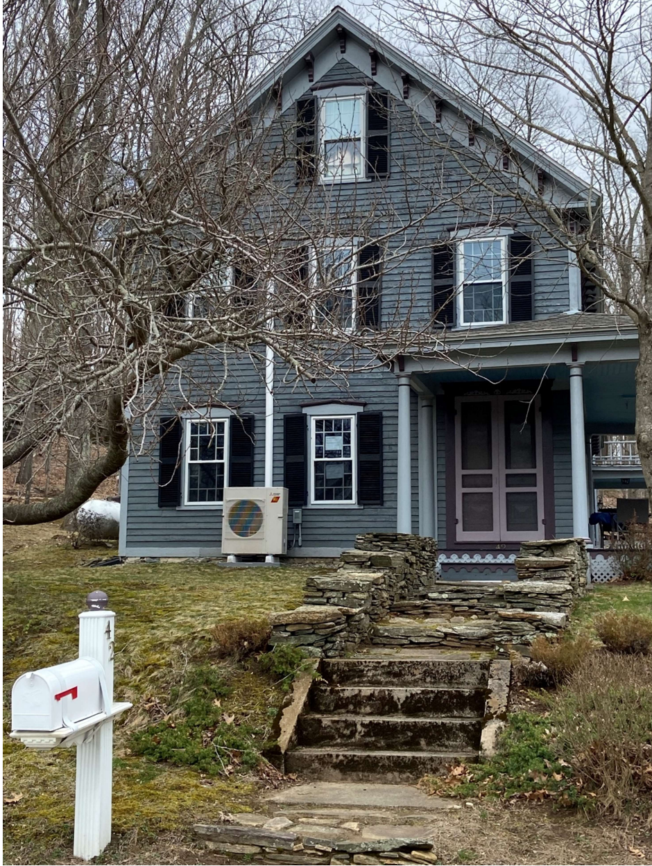
Mini split to be screened with lattice and climbing rose bush
