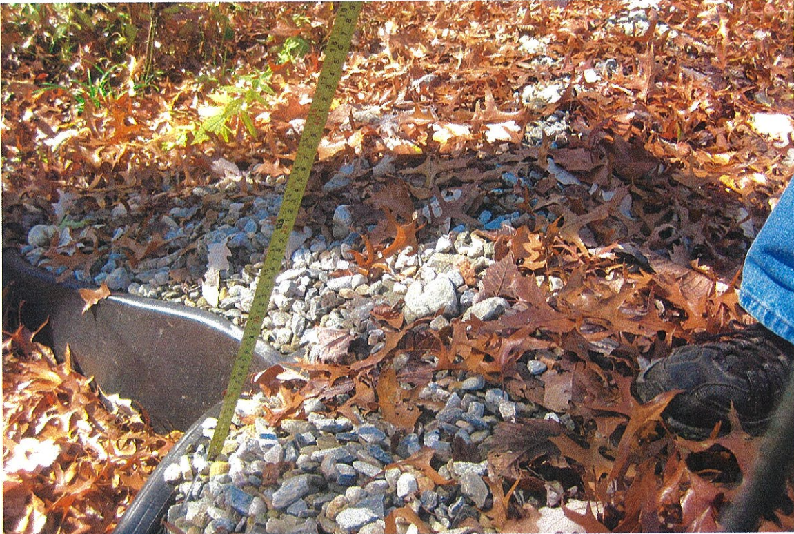
Tape measured 9" of fill over third pipe in middle crossing (westernmost pipe)
