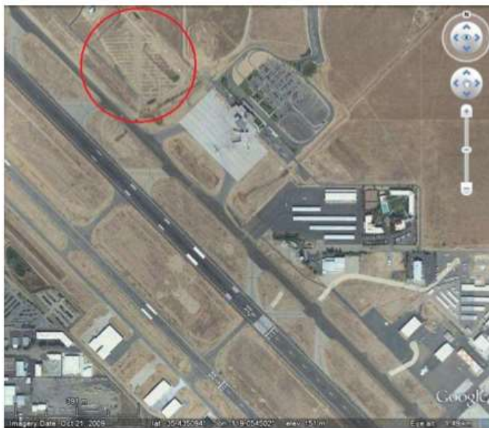
Figure 7: Bakersfield Airport showing location of solar array
